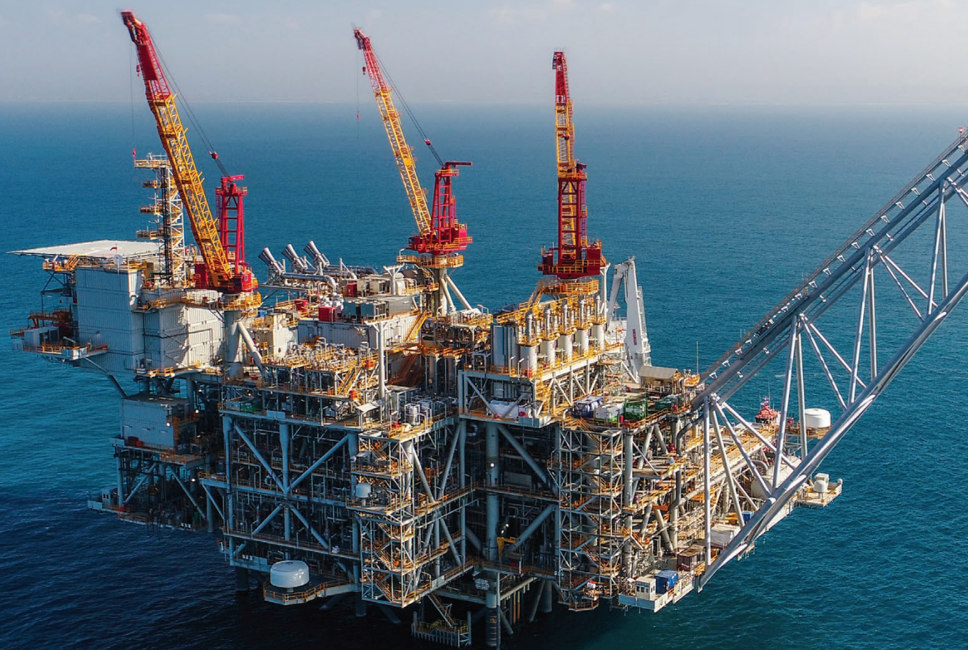
Photo: Leviathan natural gas platform, offshore Israel.
